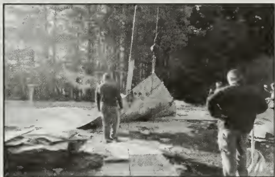
Above: (L) Existing roof membrane, underlying fiberglass insulation and old built-up roof were removed (R) The gypsum deck was very deteriorated along the rear edge and was completely removed.
